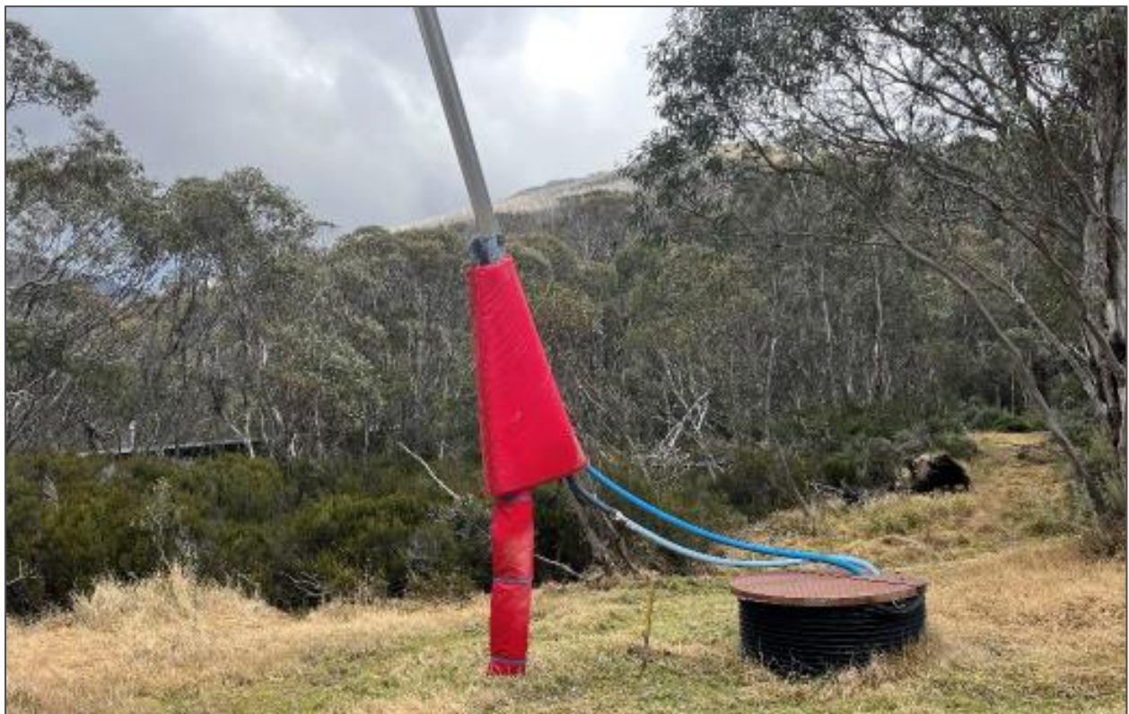
Figure 6 | Example steel pit and lance type snow gun to be replaced (Source: Applicant's Documentation)
